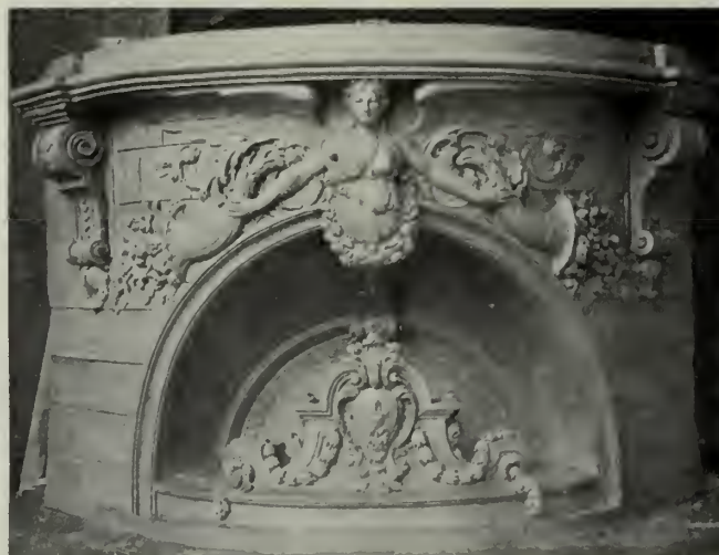
DETAIL OF CORNER ENTRANCE TO BANK BUILDING. Northwestern Terra Cotta Company, Makers. Diboll, Owen & Goldstein, Architects.
